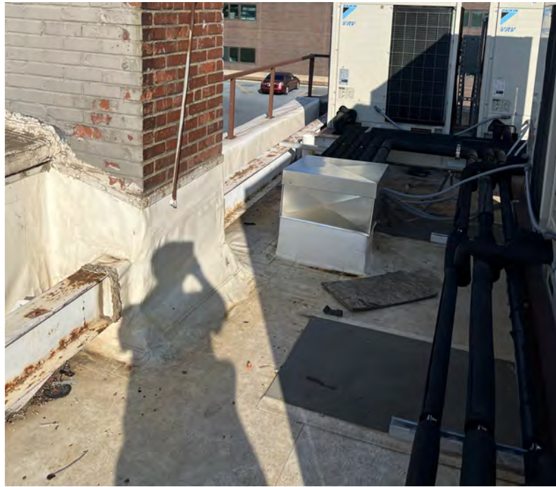
CHIMNEY TERM BAR & FLASHING 17
